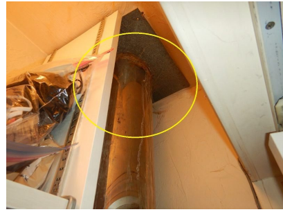
First Floor Interior Closet
